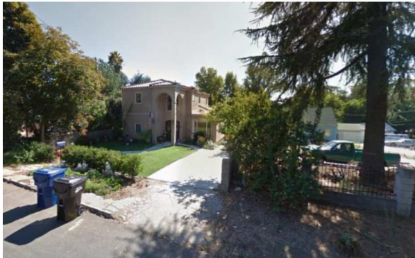
Photo No. 3 – Las Flores - Looking South
