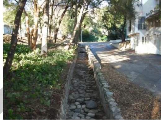
Photo No. 12 – "U" Drainage Channel looking North
