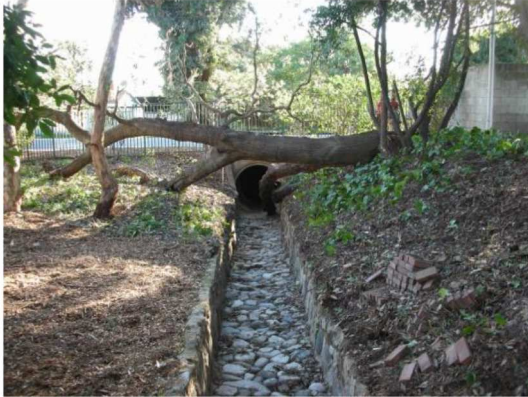
Photo No. 11 – "U" Drainage Channel looking South
